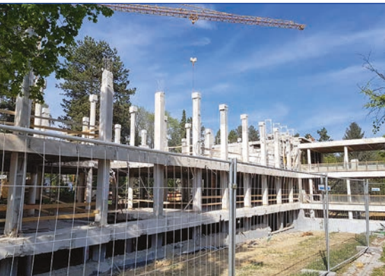
The partially-completed new building at CALT.
